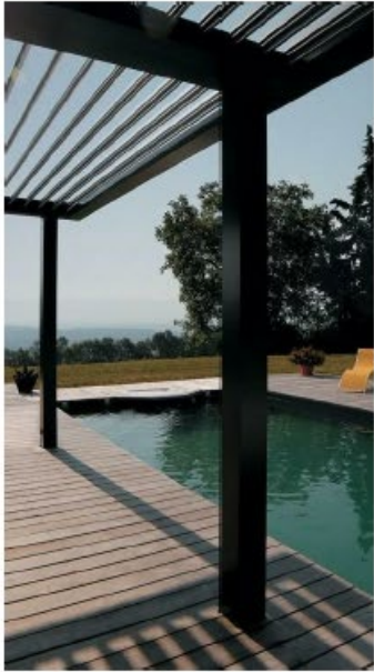
Steel pergola with operable louvres
