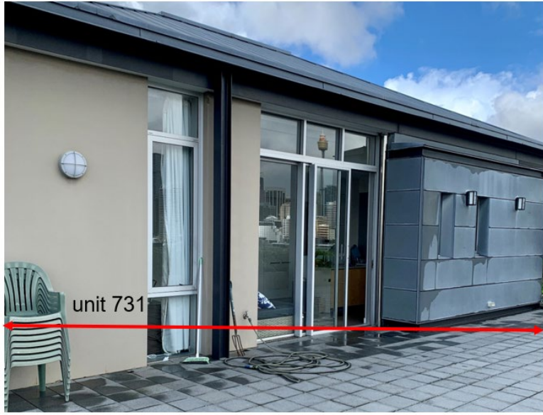
south elevation of unit 731
