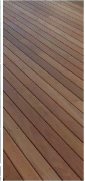
Decking to terrace
