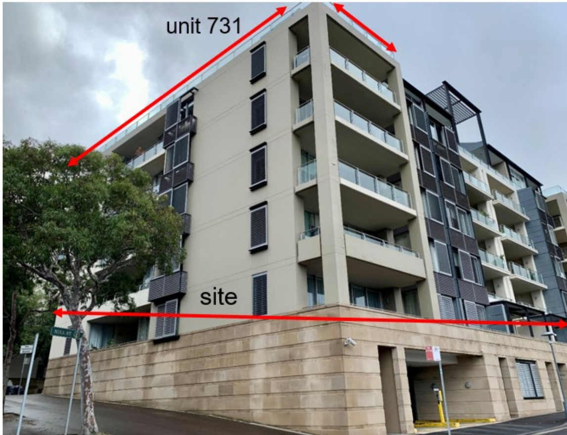
corner of Bayview Street and Mill Street
